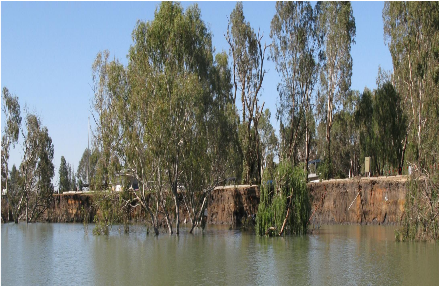
More bank collapse and cracking
