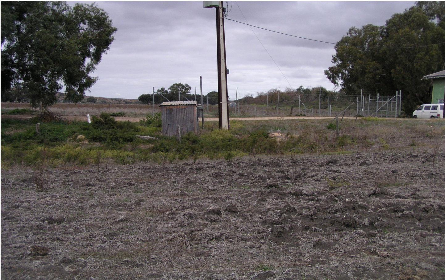
Large cracks in once laser levelled irrigation swamps
